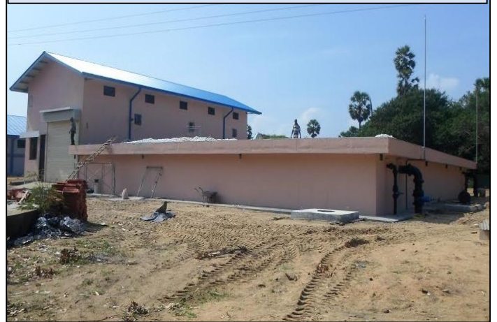
Eluthor Sum and Pump House
