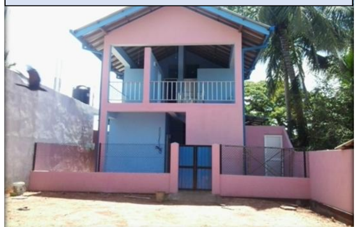
Public Toilets Stage 1 Vavuniya
