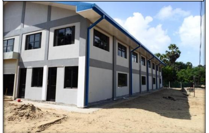
Eluthoor – Store construction
