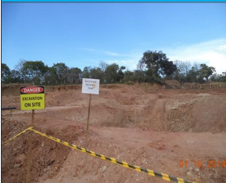
Water Treatment Plant -Excavation
