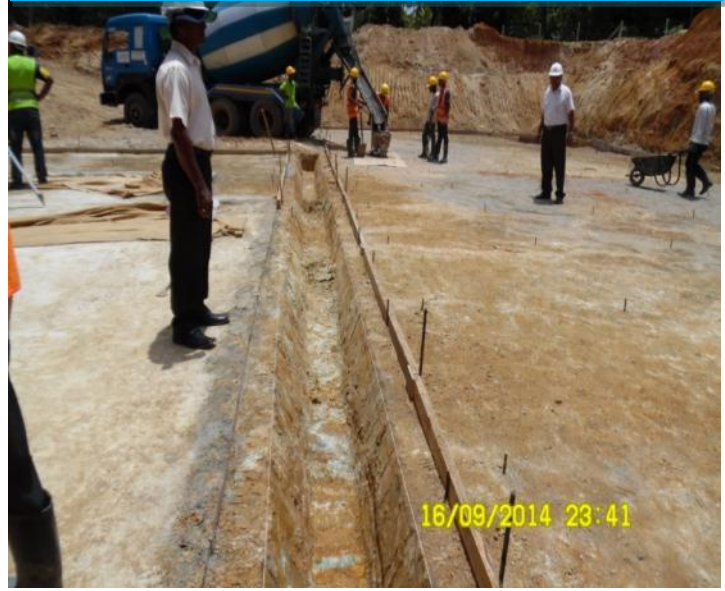
Screed concrete at clear water tank
