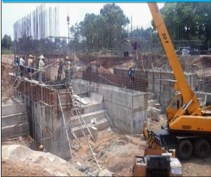
Spillway Construction
