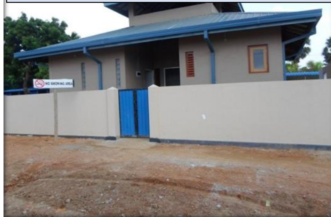
Public Toilets Stage 1 Mannar
