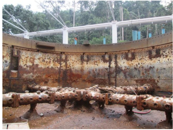
Demolished filter at Labugama
