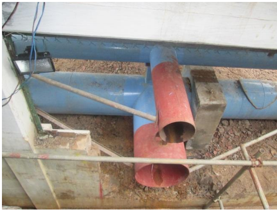
Ready to connect by-pass line at Labugama
