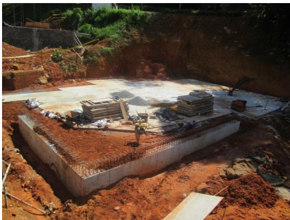
Basement for DAF Unit at Kalatuwawa
