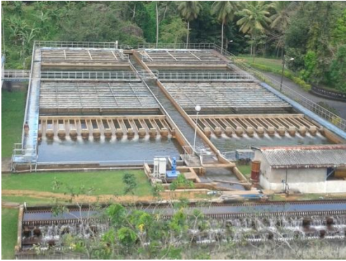
Existing Treatment Plant at Kalatuwawa
