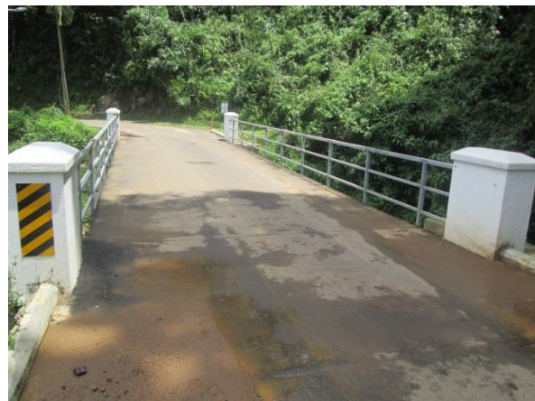
Completed Baily Bridge at Labugama
