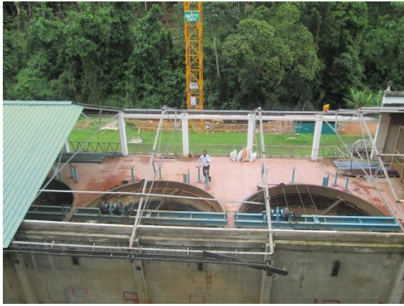
Starting demolition of Filters at Labugama
