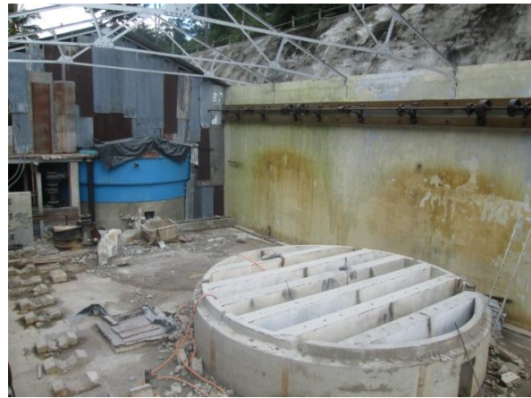
Demolished Filter Deck at Labugama
