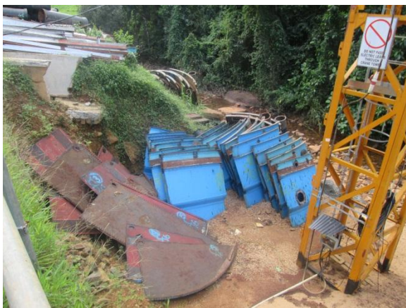
Demolished Materials near the Tower Crane
