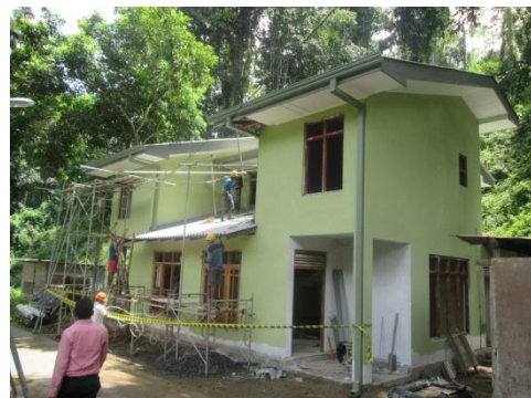
Nearly finishing of Quarters
