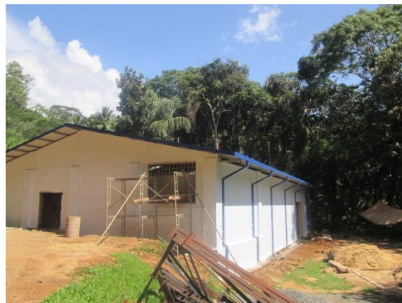
Nearly finishing of Stores Building at Kalatuwawa
