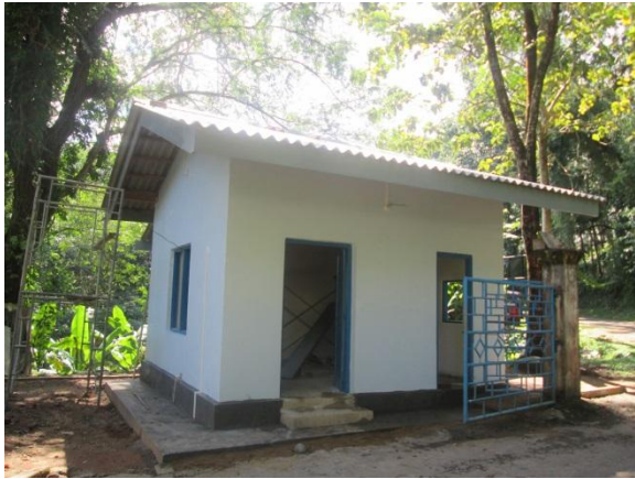
Renovated Security Room at Kalatuwawa
