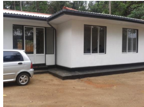
Newly Constructed Project Office at Kalatuwawa
