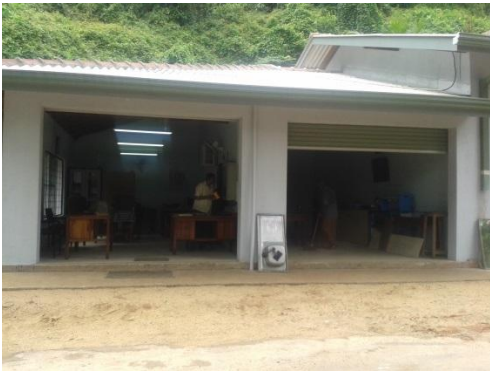
Renovated Store Building at Labugama
