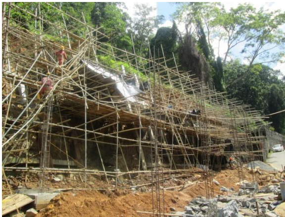
Slope establishment for Chlorine Building at Labugama
