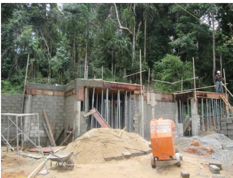
New Quarters being construction
