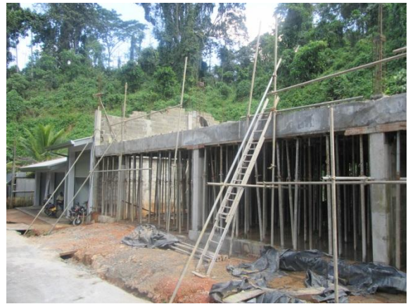
Admin Building being construction at Labugama
