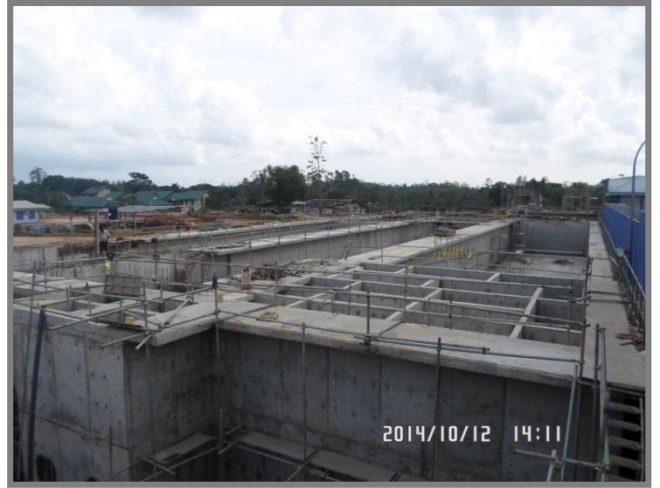
Construction of Sedimentation tank
