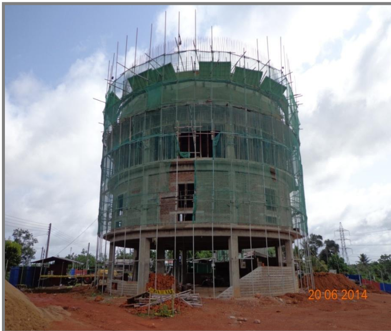
Construction of 1000 m3 capacity water tower at Welmilla
