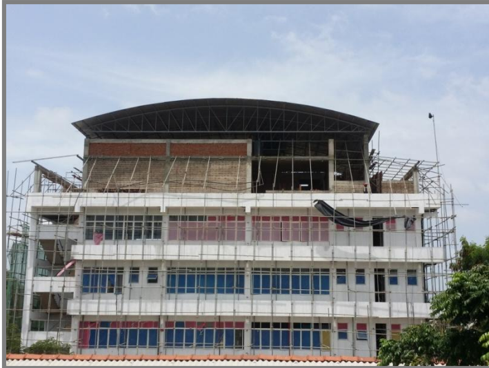
Construction of office building for RSC (W/S)
