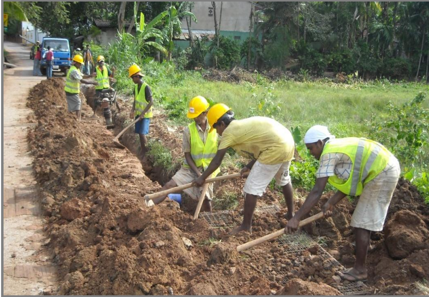
Pipe laying along a P.Sabha road
