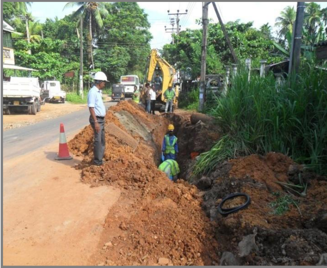
Pipe laying along a UC road
