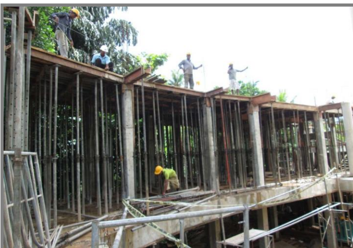
Construction of Area Engineers Office Building - Piliyandala
