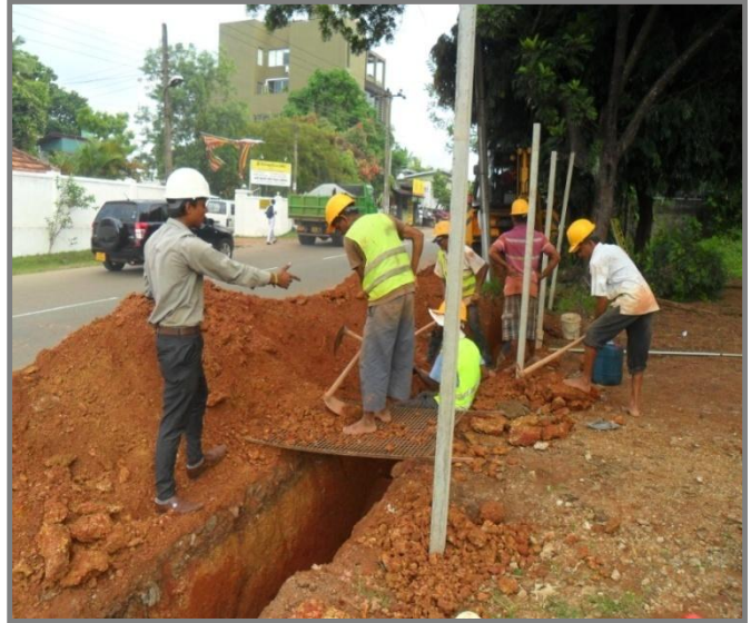
Pipe laying along Kesbewa – Pokunuwita road
