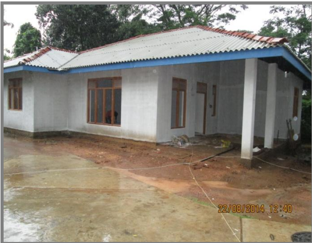
Construction of OIC's office - Kumbuka
