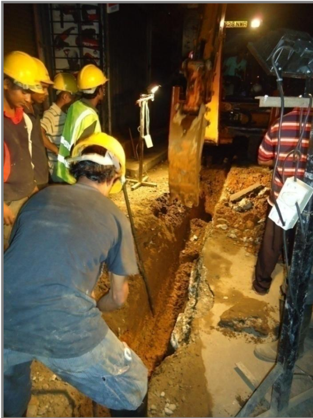
Pipe laying at Abdul Hameed Street
