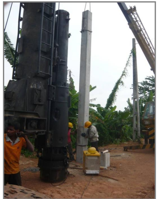
Concrete pile driving for pipe laying in marshy area -2 (Kahatawela-K/B road)
