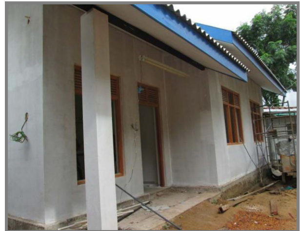
Construction of quarters for OIC - Kumbuka
