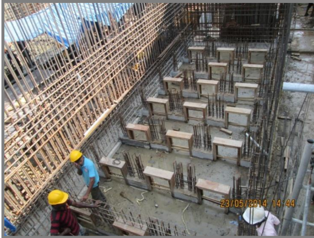
Construction of Filters
