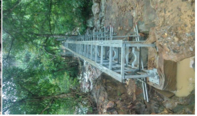
Steel Bridge for Raw water Main
