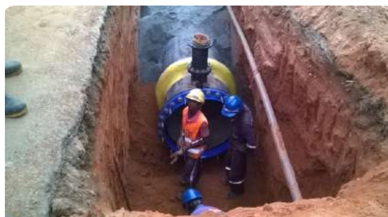
Fixing of air valve along 1000 mm dia DI Transmission Main
