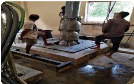
Pumps installation
