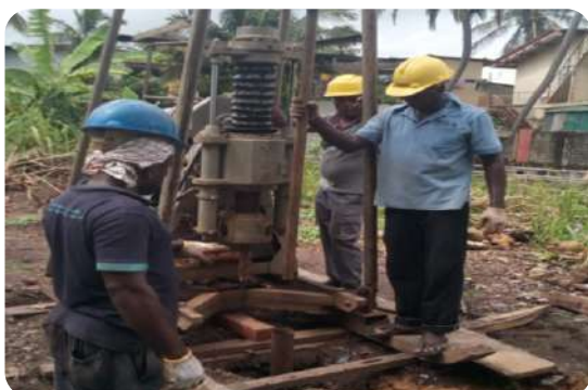
Soil Investigation Work at Pump Station Lands
