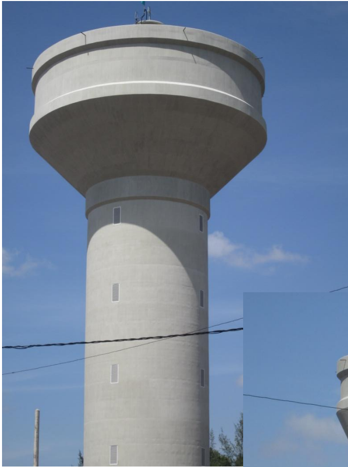
Kilinochchi Elevated Water Tower (1000m 3 )
