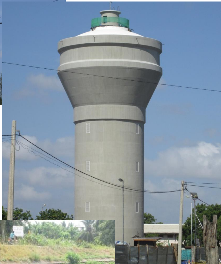
Paranthan Elevated Water Tower (450m 3 )
