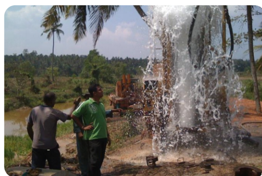
Well construction for groundwater dev. for Minuwangoda WSS
