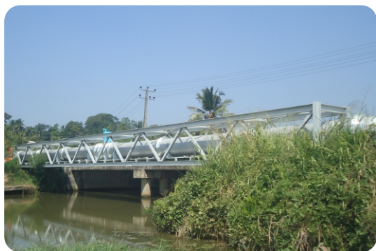
Pipe bridge at Kahatawela (Kesbewa-Bandaragama Road)
