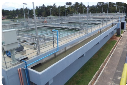
Sedimentation & Flocculation Basins
