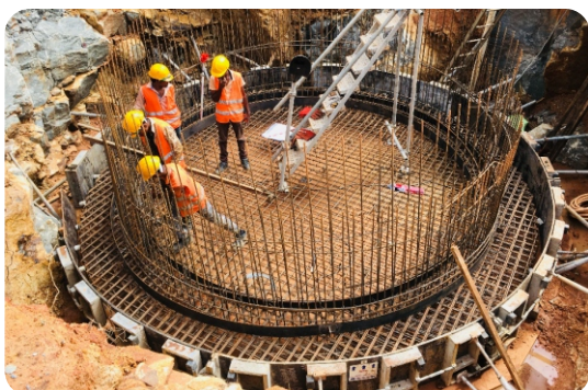
R/F & F/W fixing work for Sludge Thickener Base at WTP Sulugune
