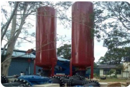
Surge vessel installation at Baddegama WTP
