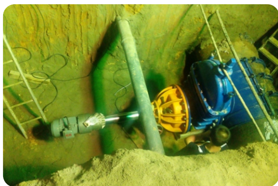
Hot Tapping Process at Godagama Junction
