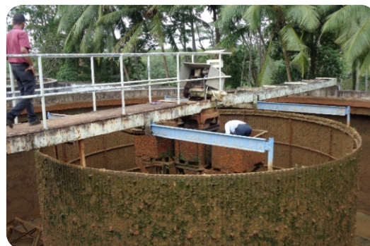
Rehabilitation of Existing Clarifier at Kethena
