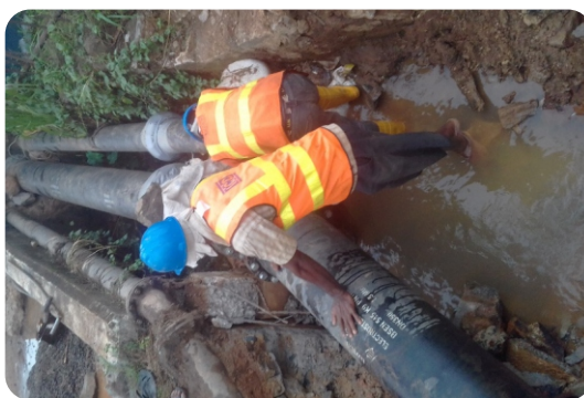
Pipe line culvert crossing
