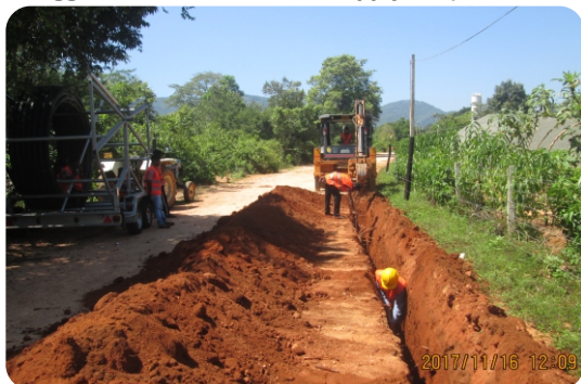
Pipe Laying Work
