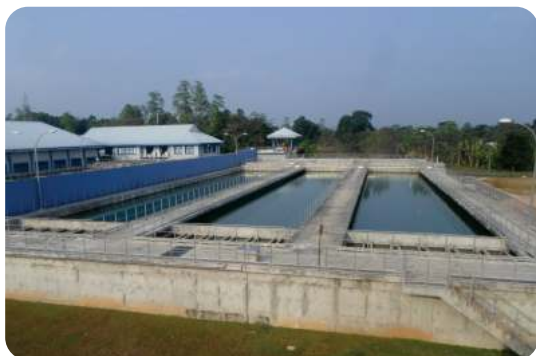
Completed sedimentation tanks and collecting channels
