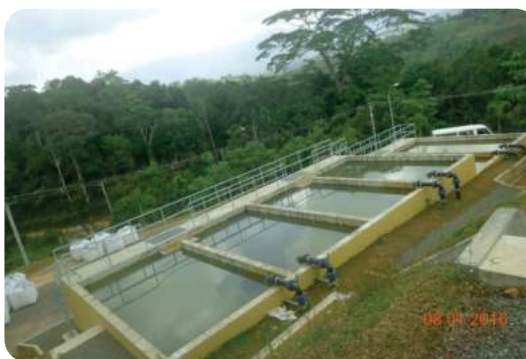
Water Treatment Plant - Balangoda
