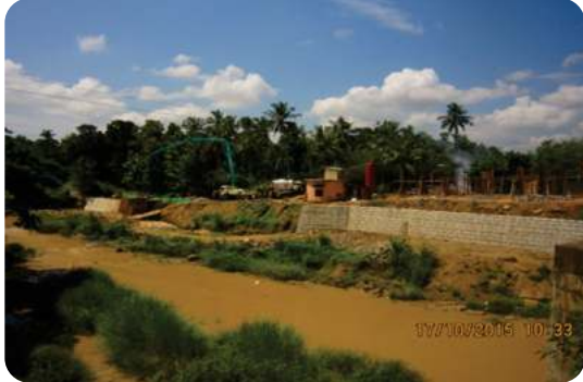
Construction of Retaining wall of the Intake and Pump House
