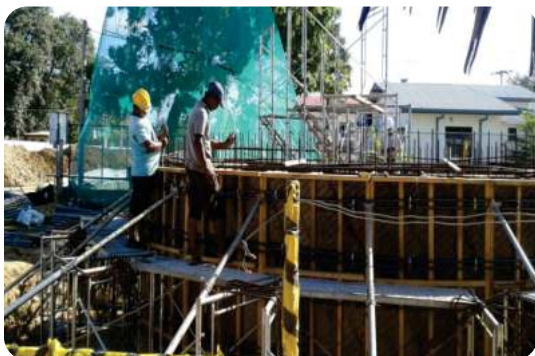
Tower construction at Velanai
