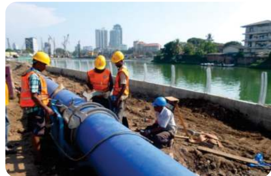
630 mm HDPE pipe laying at Jhone Keels Site (Slave Island)
