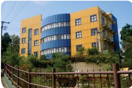
Regional Support Center Building at Kadawatha
