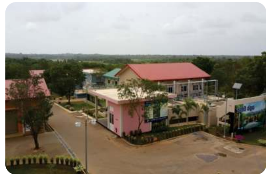
water treatment plant at Ruhunupura WSP
