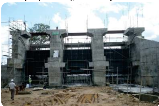
Spillway Structure Under Aru Dam construction in Vavuniya
