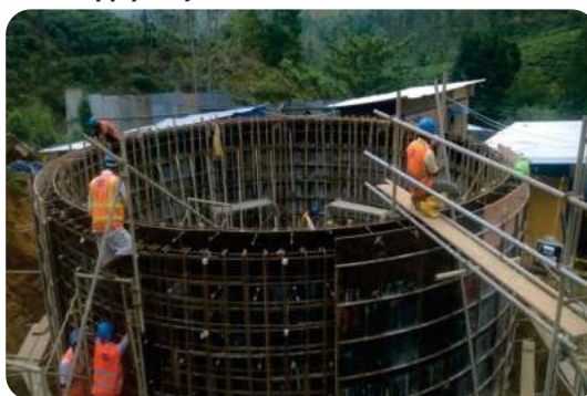
Construction of wash water recovery tank
