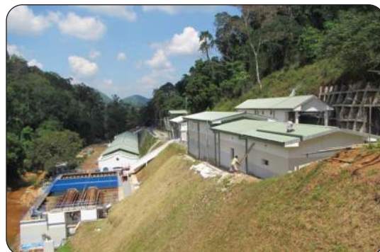
Construction of water treatment plant at Demodara
