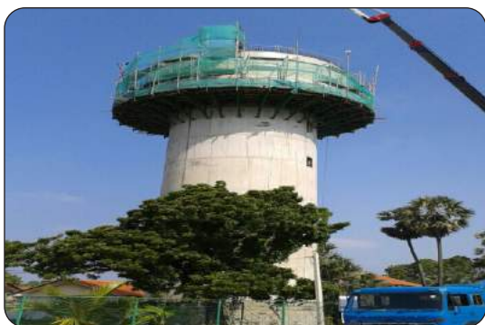
Water Tower at Velanai
