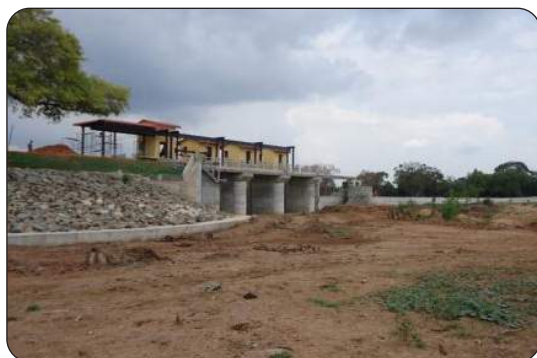
Spillway Structure NeroPer-Aru Dam construction in Yavuniya
