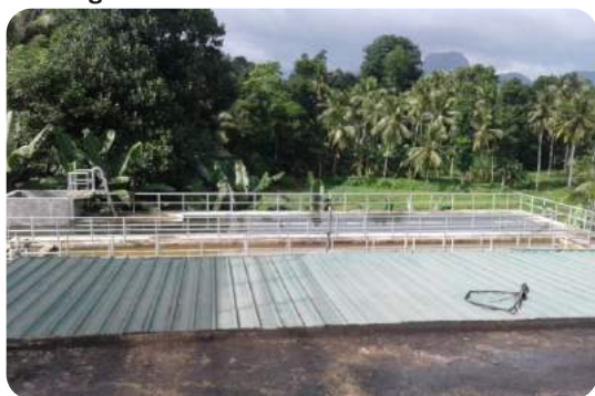
Mawanella treatment plant
