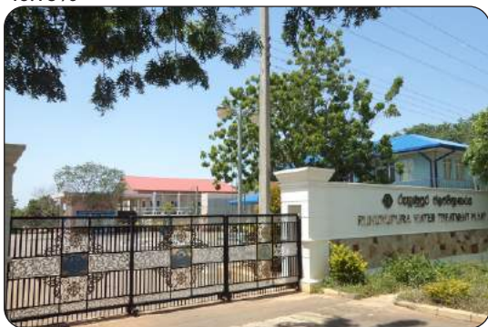
Ruhunupura Water Treatment plant
