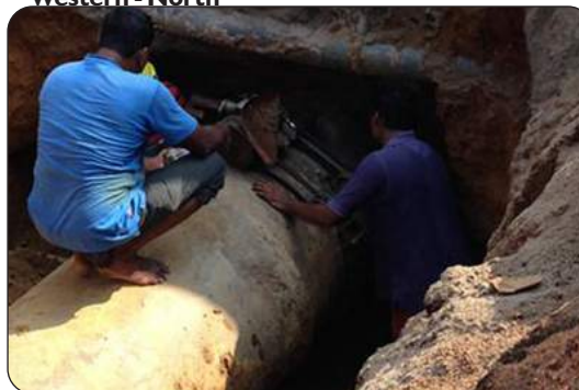
Biyagama - Mabima pipe laying work
