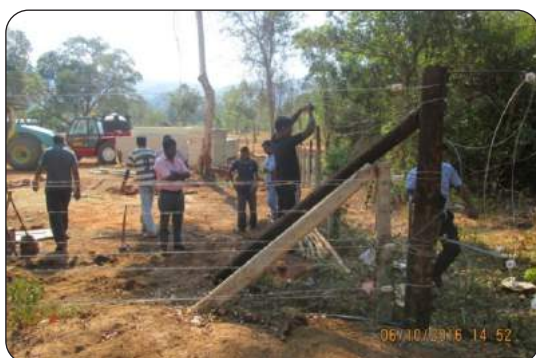
Elephant fence arranged for Contractor's main yard
