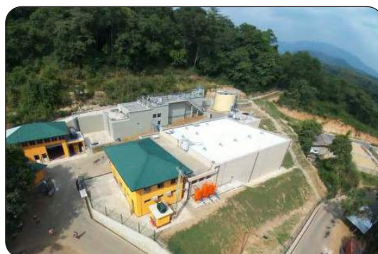
Kumbukkana treatment plant
