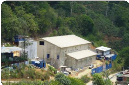
Labugama Water Treatment Plant
