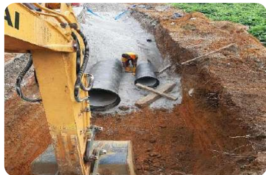
Laying of raw water and clear water pipe lines in one trench
