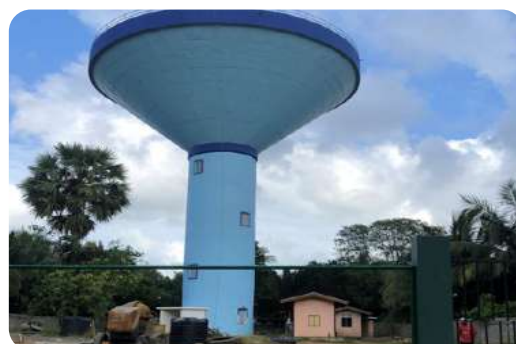
Serunuwara Tower Construction
