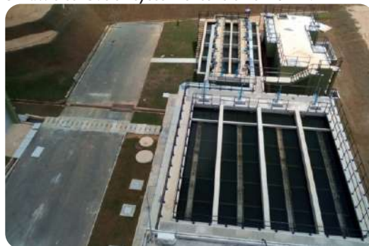
Puttalam Water Treatment Plant
