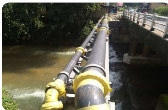
Pipe laying across the Bridge No. 53/3, Avissawella
