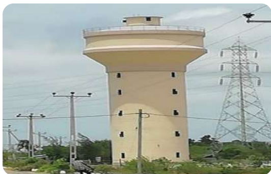
Completed Water Towers
