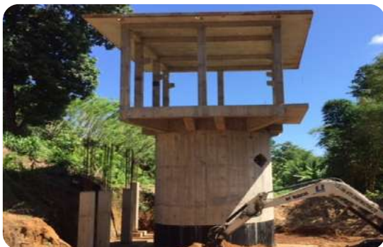
Intake Well and Pump House
