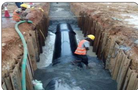
Orugodawatta Pipe Laying
