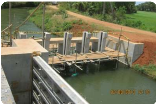
Ruhunupura Water Supply Project - Construction of Control Gate
