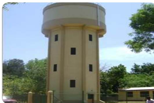
Kataragama WSS - 225 cu.m Capacity Water Tower
