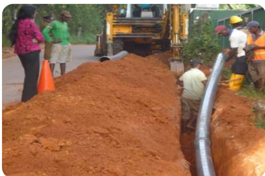
Laying of uPVC pipes along Rathupaswala - Nedungamuva road
