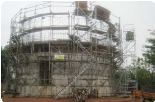
Construction of Mahaweli Water Tower (2,000 cu.m)-Ruhunupura
