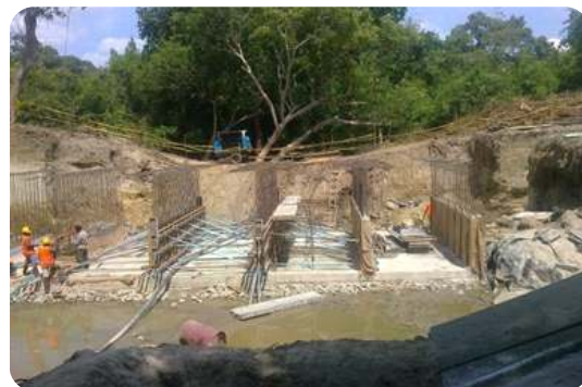
Surface Water Development in Vavuniya Causeway Construction
