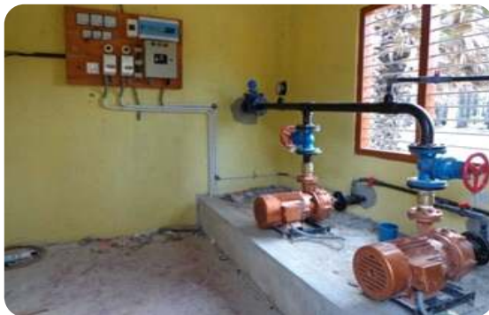
Rehabilitation of Velanai Pump House
