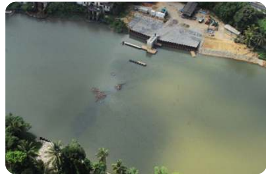
Semi Permanent Salinity Barrier at Ambatale
