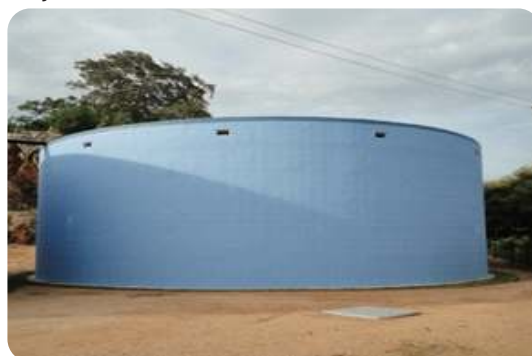
Construction of 2,000 Cu.m. capacity ground reservoir at Wellamandal
