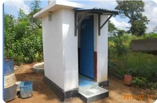
Latrine construction in Hambantota district
