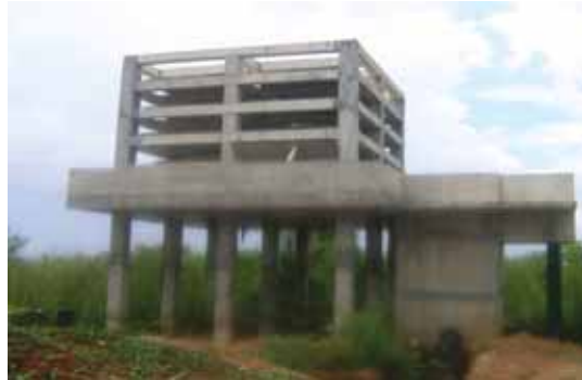
Construction of Aerator of Thihagoda Water Treatment Plant
