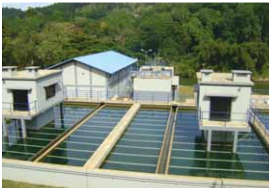
Meewathura Water Treatment Plant
