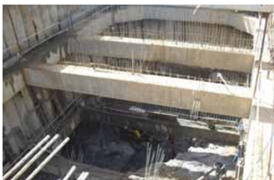
Construction of Wellawatte New Pump House
