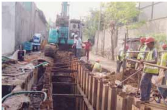
Pipe laying in Kandawala Mawatha
