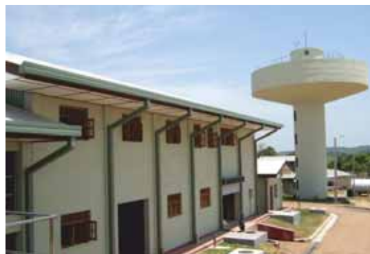
Ampara Treatment Process Building
