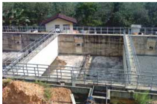
Construction of Slow Sand Filter at Udugama WTP
