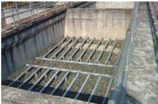
Construction of Roughing Filter at Radampola WTP
