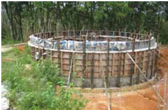
Construction of Roughing Filter at Pitabeddera WTP
