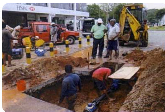
Installation of Boundary Meters
