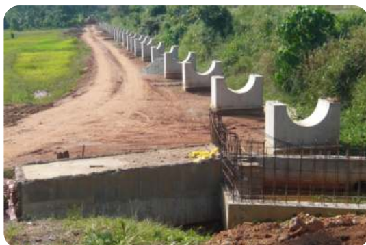
Pipe supports at Gammanpila tank bund area for exposed pipes
