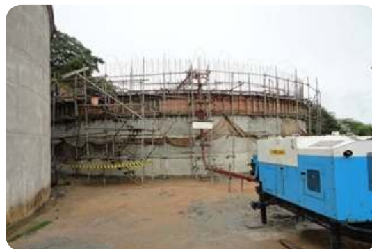
Construction of 2000 Cum capacity ground reservoir at Wellamanal
