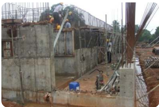
Erection of Reinforcement for Rapid Sand Filter
