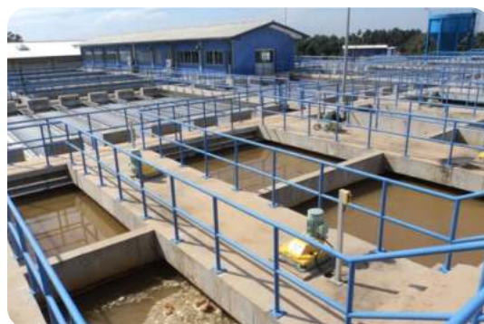
Flocculation & Filtration Tanks
