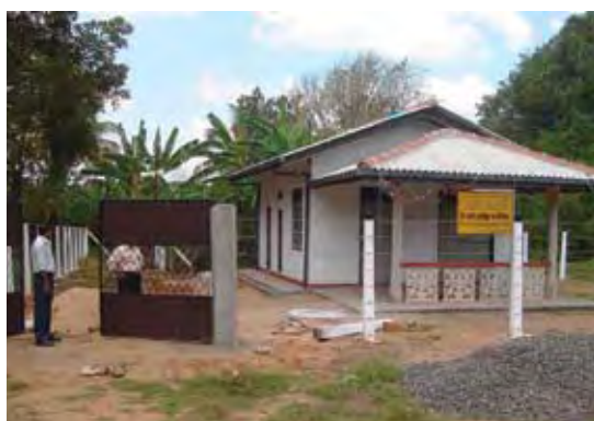
Pump House Galwanguwa - Ipalogama
