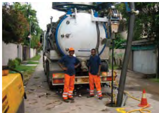
Cleaning of Sewer Line
