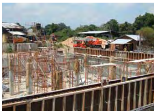
Ampara Clear Water Tank
