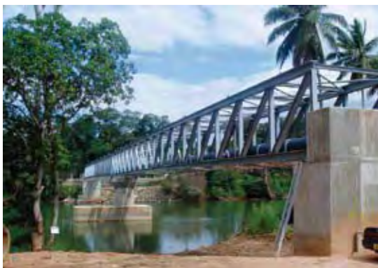
Mahaweli Pipe Bridge for Kandy
