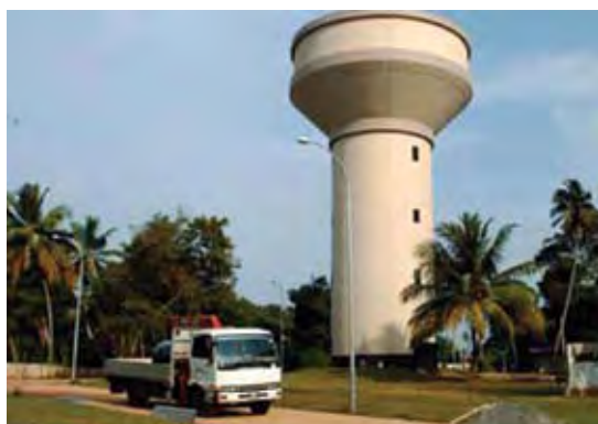
Kakkapalliya Water Treatment Plant
