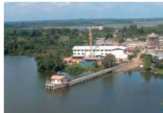
Ampara Intake Bridge
