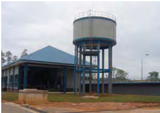
Overhead Tower - Plant Water System
