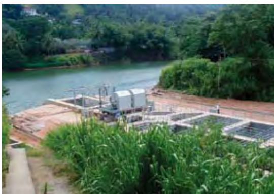
Construction of Intake for Kandy
