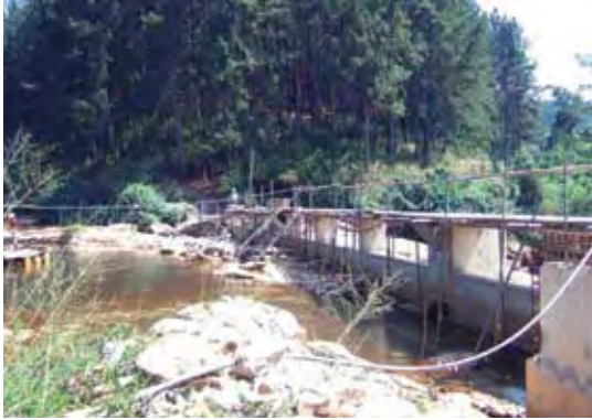
Nawalapitiya Intake Dam
