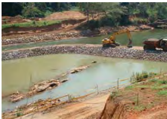
Establishment of Cofferd Dam
