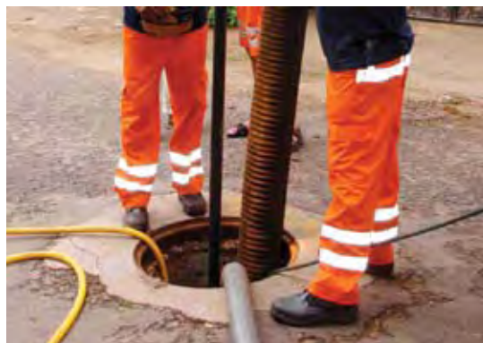
Closer View of Sewer Cleaning Process
