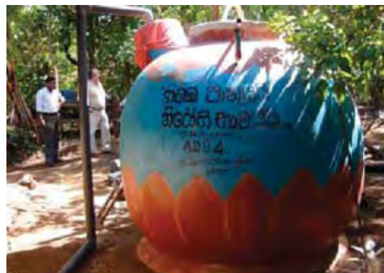
Completed Rain Water Harvesting Tank at Anuradhapura
