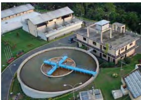
Galle Water Treatment Plant
