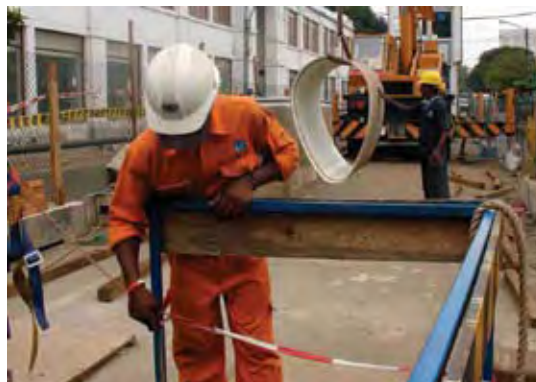
Lining Sewer Lines
