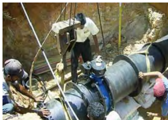
Hambantota Pipe Laying
