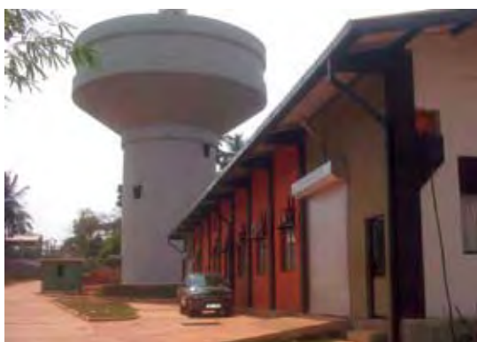
Mahara Tower, Reservoir and Pump House
